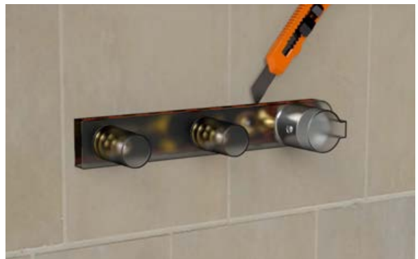
4. Once tiled it is easy to remove the protective case with a sharp blade
